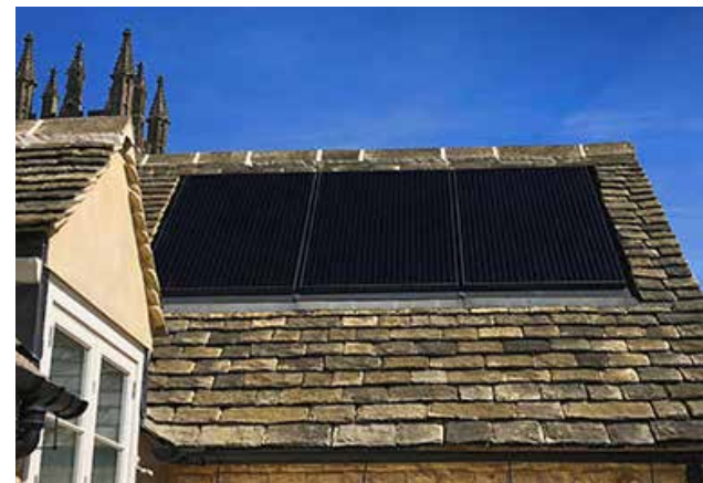
Figure 20: Example image showing the use of solar panels in traditional buildings by making them flush with the tiles and creating contrast.
