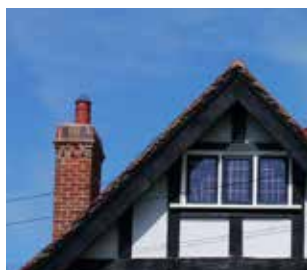
Gable ended roof
