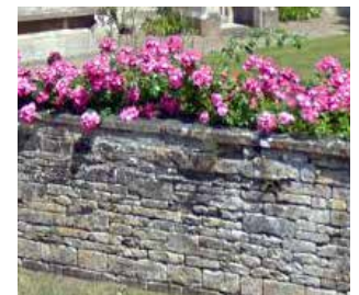
Dry-stone wall with flat top
